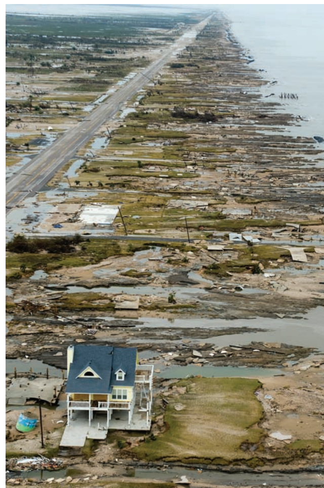
FIGURE 6.21 Damage from Hurricane Ike in 2008. Hurricane Ike, which made landfall in Gilchrist, Texas, was the third most destructive hurricane to ever make landfall in the United States.
