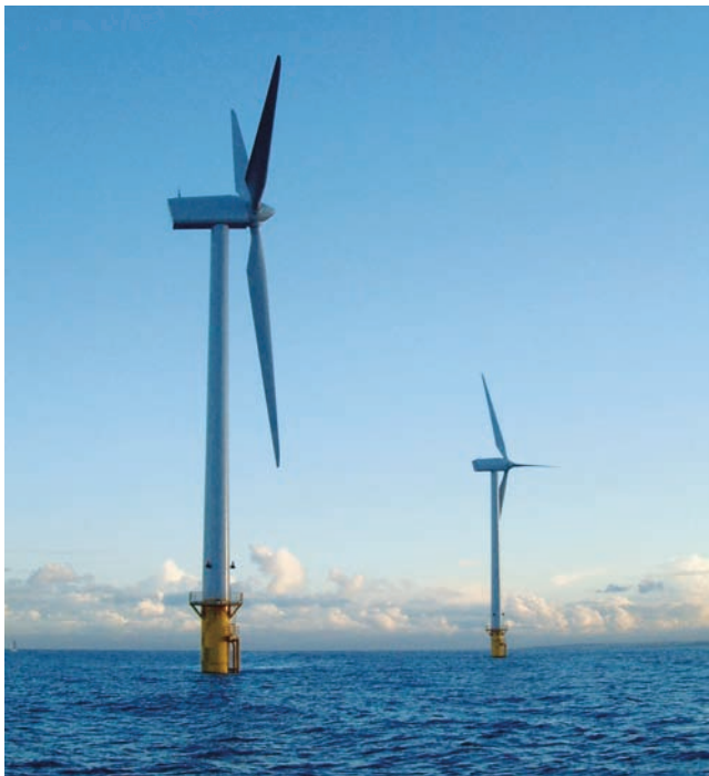
FIGURE 6.26 Offshore wind farm. Offshore wind turbines form a part of a wind farm in the North Sea off the coast of Blyth in the U.K.
