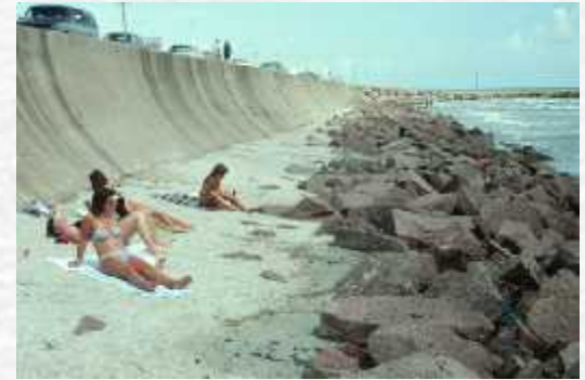
Beach loss eventually occurs in front of a seawall for a beach experiencing net longterm retreat.
